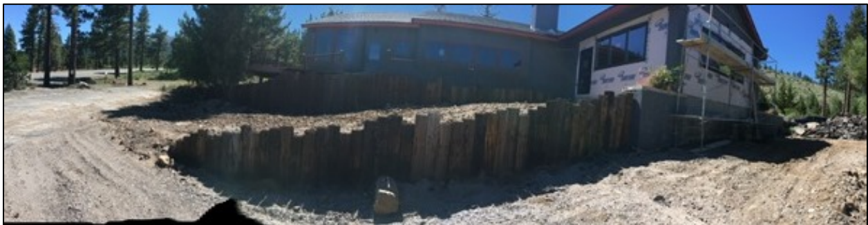
Looking northwest at existing structure (currently being remodeled)
